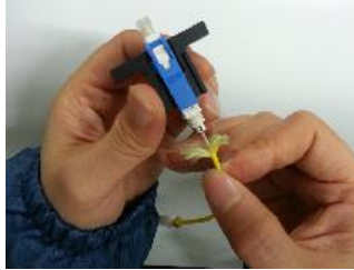
2/ Insert the cleaved fiber slowly into the rear of connector until connection is made.
