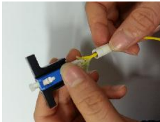
4/ Divide Kevlar into 2 equal portions and screw the lock nut onto back of connector to secure Kevlar tightly. Then, slide the boot up. (If for 250 or 900µm cable, jump to point 5)
