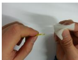
7/ Clean the stripped fiber with alcohol wipe to remove any debris.
